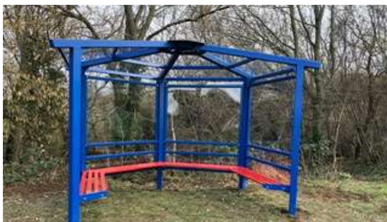
A new Youth Shelter located at Kings Stanley Playing Fields, delivered by the Parish Council using Neighbourhood CIL funding towards the project. Delivered in February 2023.
