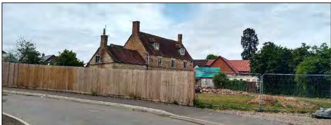
Photo 3: Image of the Listed Parklands Farmhouse (C) looking west
