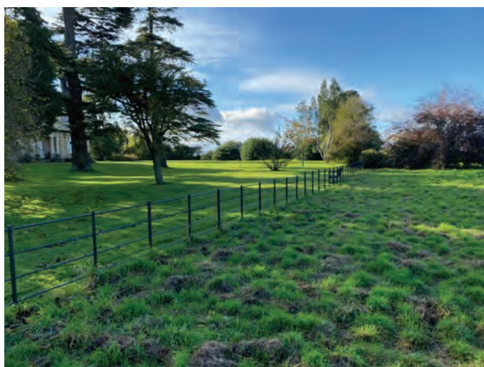
Photograph 10: Southeast boundary iron railings.
