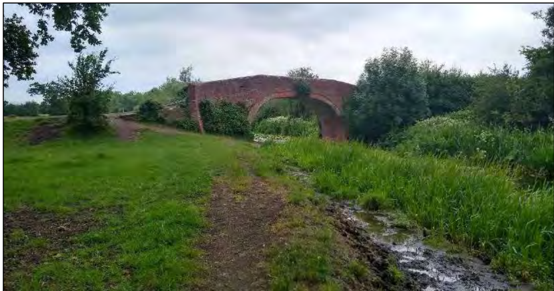
Photo 8: Image of the Bridge on the Stroudwater Canal, looking north
