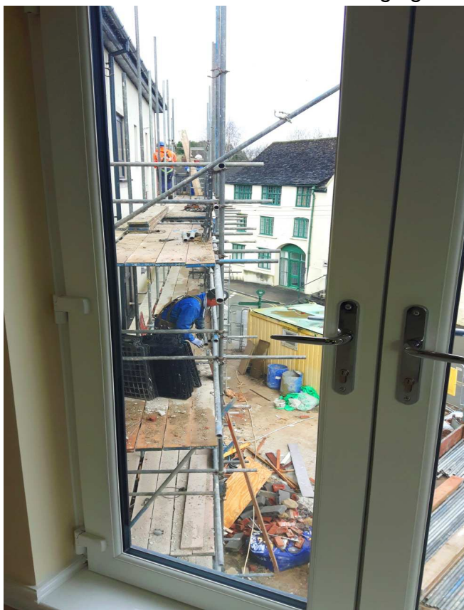
Affordable flats under construction in Dursley, 2017
