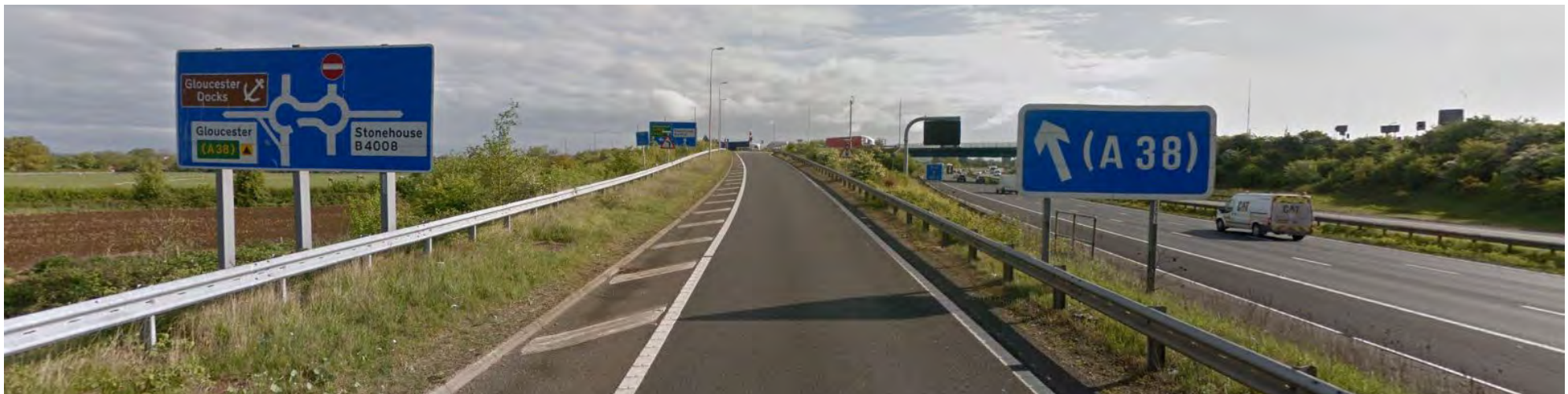
View M5 junction 12 exit slip road
