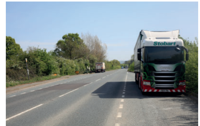
Existing A419 lay-bys bordering allocation site PS20
