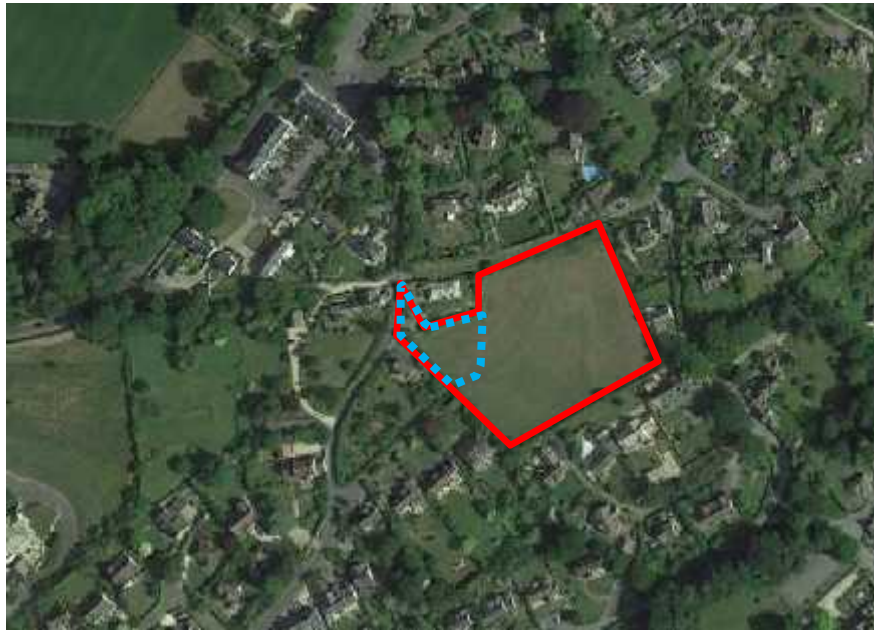
Site outlined red and application no. S.17/0792/OUT boundary outlined in blue dot on aerial photograph (For indicative purposes only)
