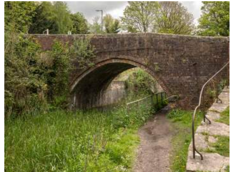
Image 51: Bridge over the Severn Thames Canal
