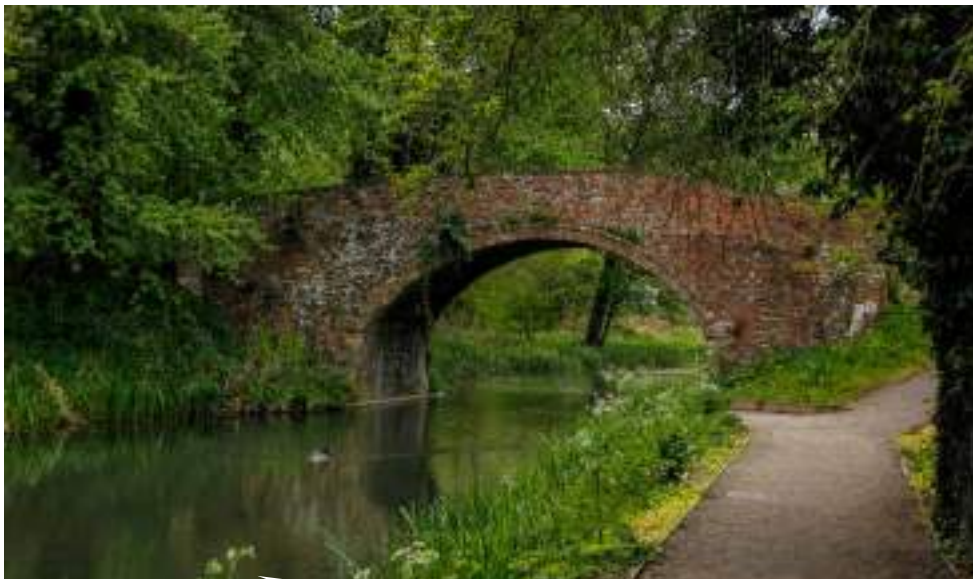
Image 30: Bridge over Severn Thames Canal
