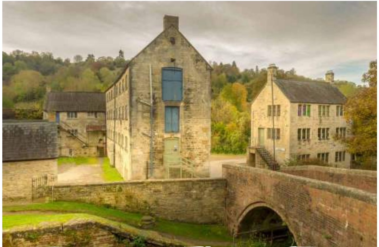
Image 14: Bourne Mills in Brimscombe
