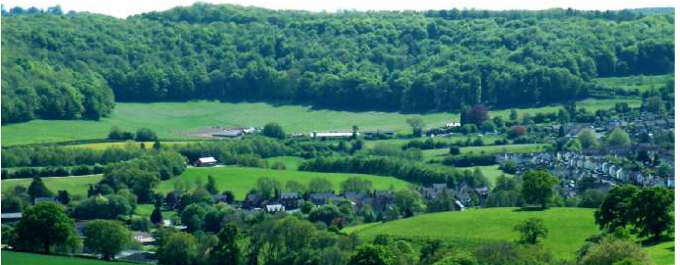
Fig B [vi] - View from Cam Peak looking towards [Pump House]
