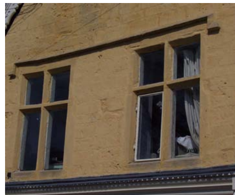
Above: 3, Middle Street, drip moulds and cross-windows
