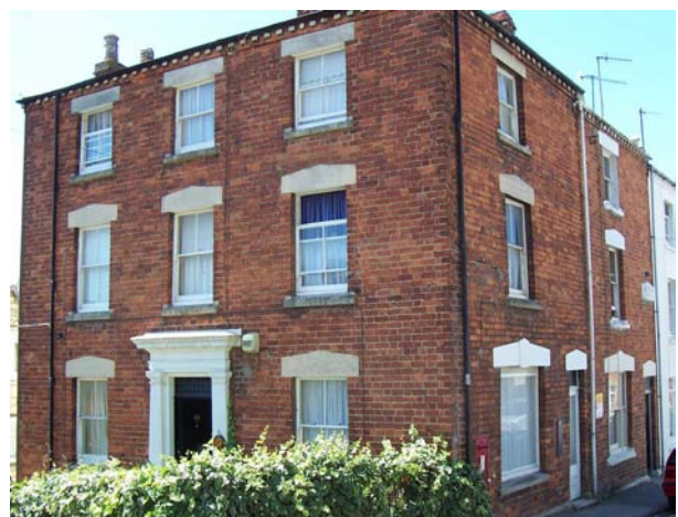
Above: 59, Middle Street; demonstrating a symmetrical arrangement of sash windows
