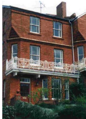
Painted iron railings add a decorative flourish to this substantial red brick property
