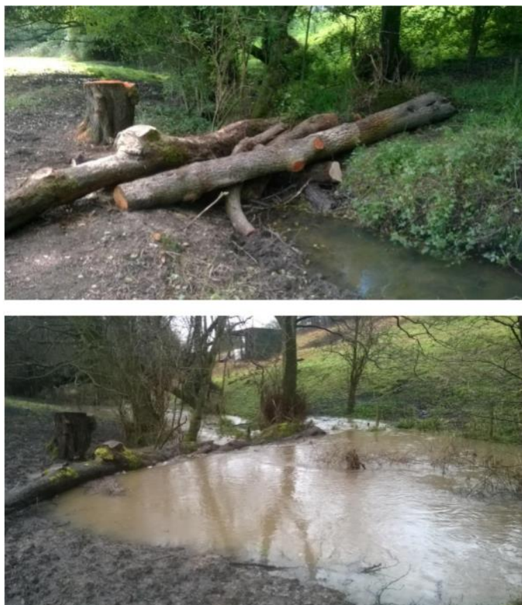
Figure 8-1: Leaky dam on Stroud Slad Farm, Slad Valley (low and peak flow in photographs) Source: Stroud Rural SuDS, Susdrain
