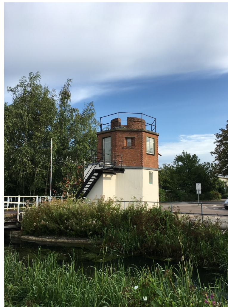
Plate 16: Grade II Listed The Gatehouse at Bonds Mill viewed from the Stroudwater Canal towpath. The asset is not visible from within the site.
