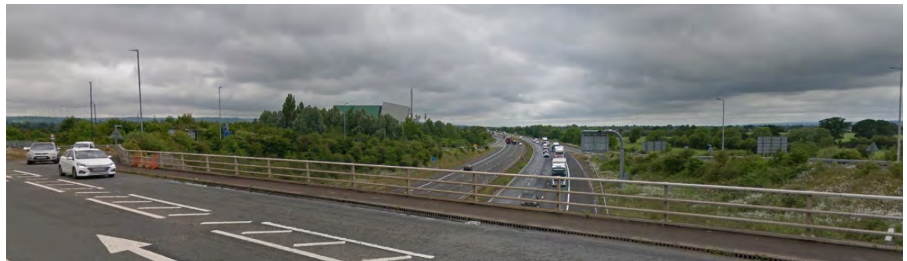
View southbound M5
