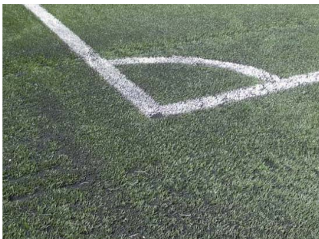
Figure 14: accumulated infill material in the corner area
