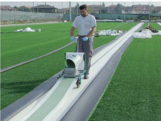
Figure 8: preparation of the seam tape
