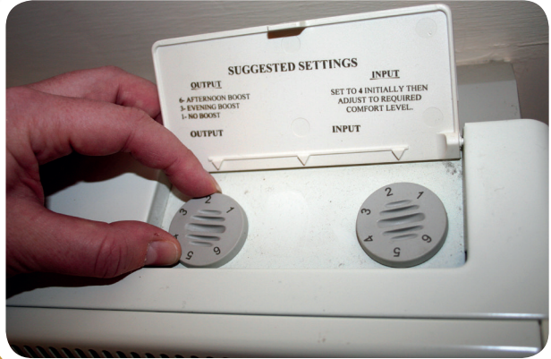
Examples of storage heater controls
