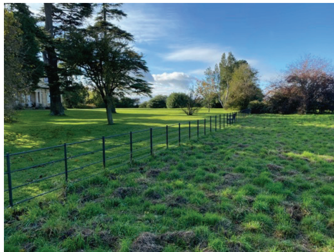
Photograph 10: Southeast boundary iron railings.
