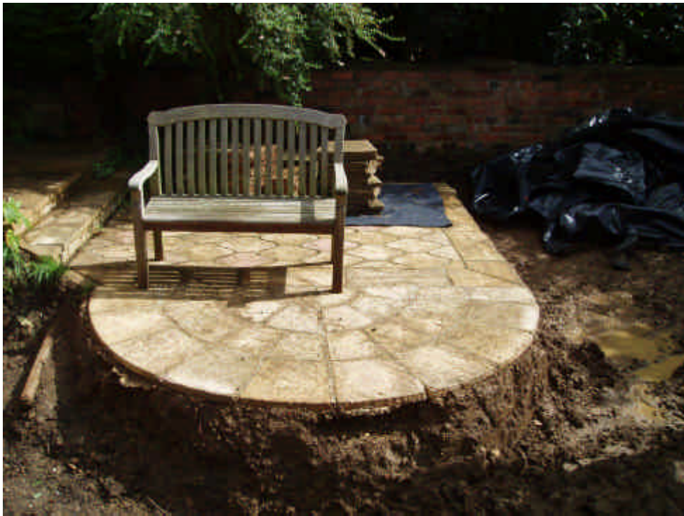
Photograph 5: Section of patio left during works (August 2008)
