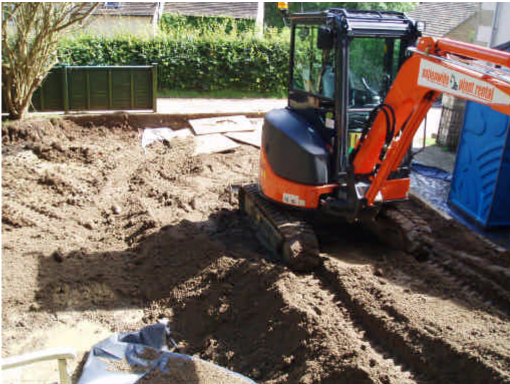
Photograph 6: Beech Cottage main garden during backfill (August 2008)
