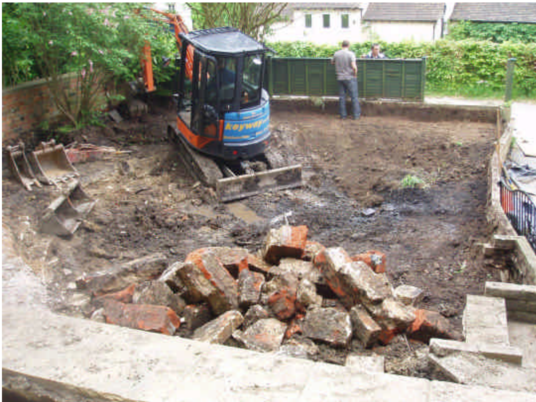
Photograph 2: Beech Cottage main garden during works (May 2008)
