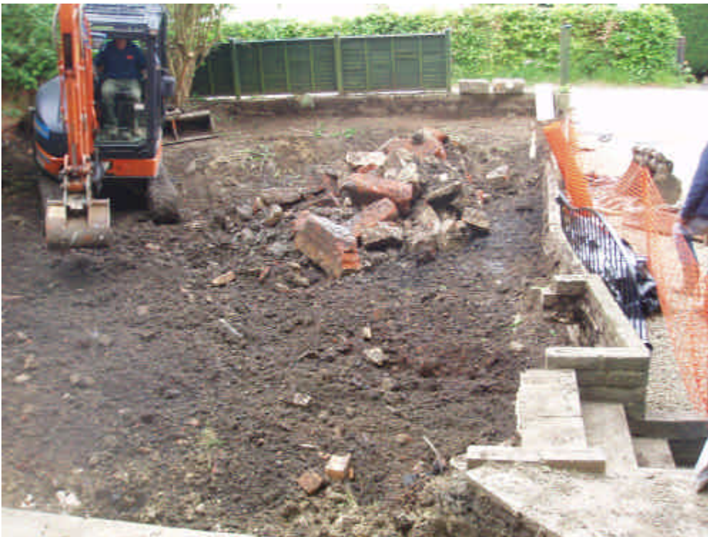
Photograph 12: View of main garden and driveway during works (May 2008)
