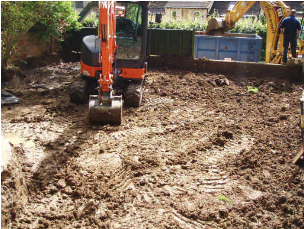
Photograph 4: Beech Cottage main garden during excavation (August 2008)
