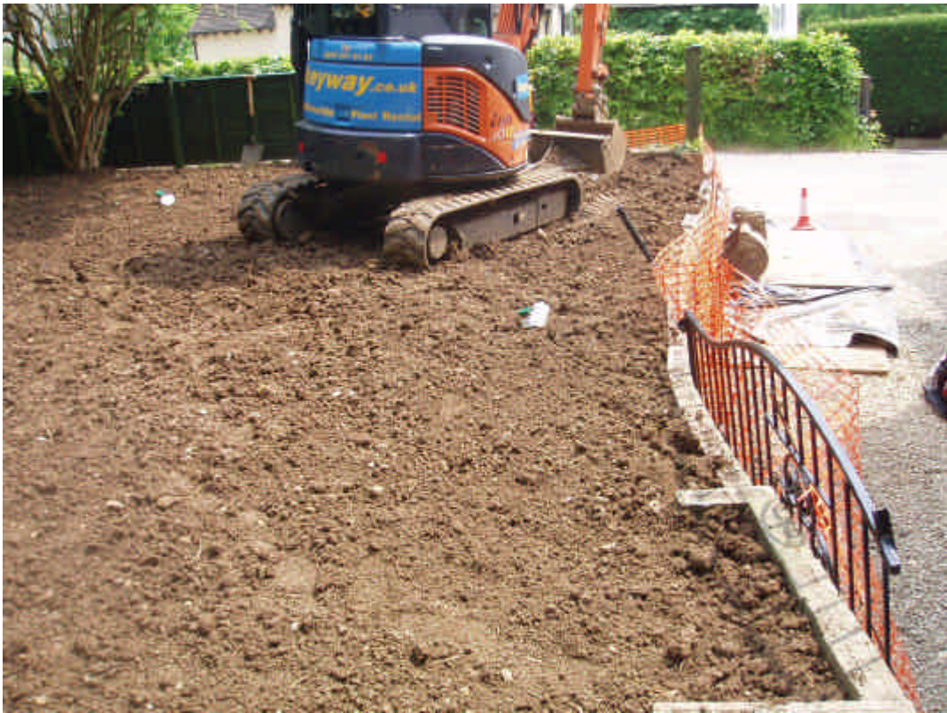
Photograph 13: View of main garden and driveway after backfill (May 2008)
