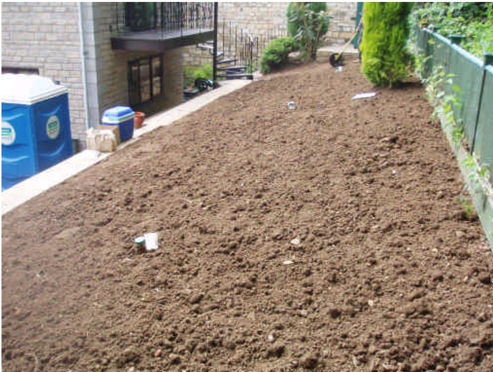
Photograph 7: Beech Cottage raised garden area after backfill (May 2008)
