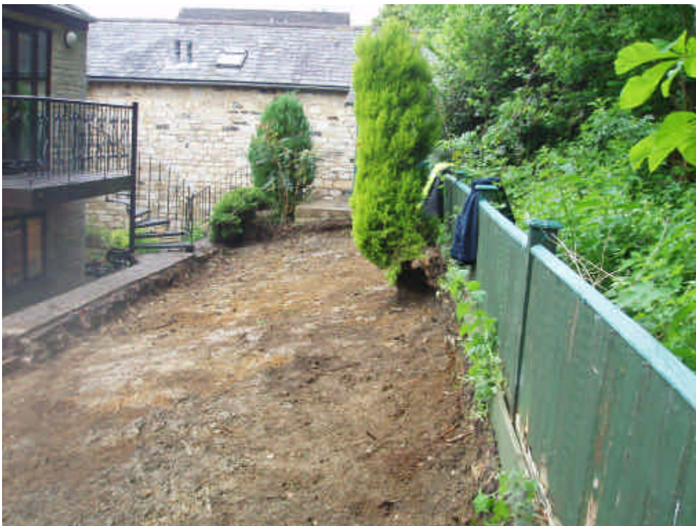
Photograph 6: Beech Cottage raised garden after excavation (May 2008)
