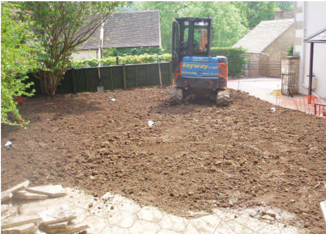
Photograph 3: Beech Cottage main garden after backfill (May 2008)
