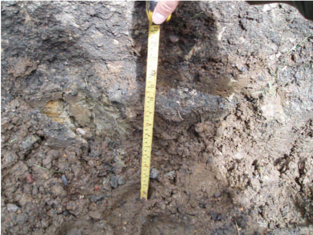
Photograph 3: Depth of excavation in main garden; 400mm (August 2008)
