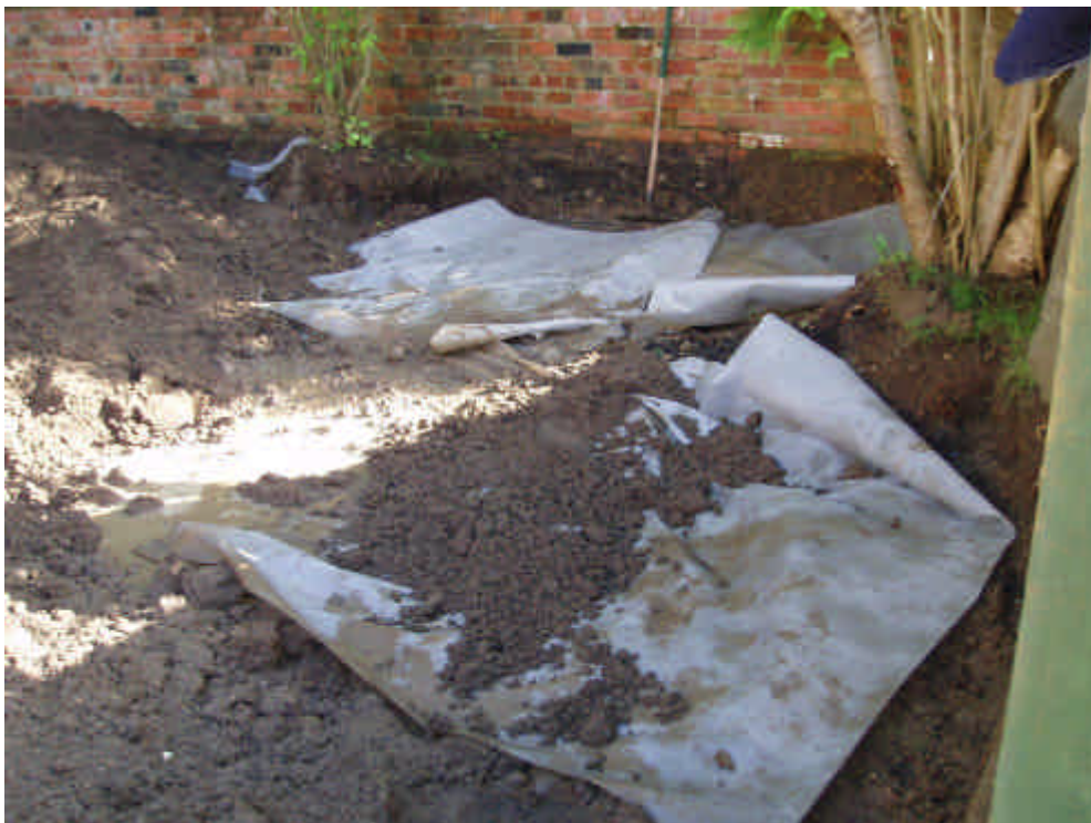
Photograph 6: New root restriction membrane installed during back fill (August 2008)
