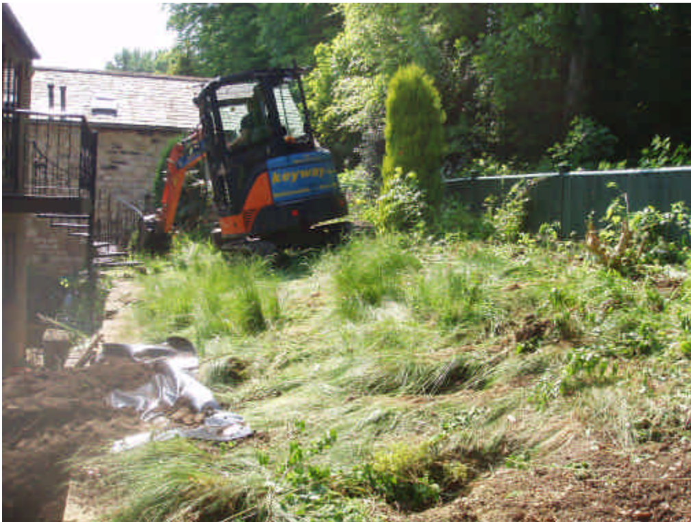
Photograph 5: Beech Cottage raised garden area during works (May 2008)
