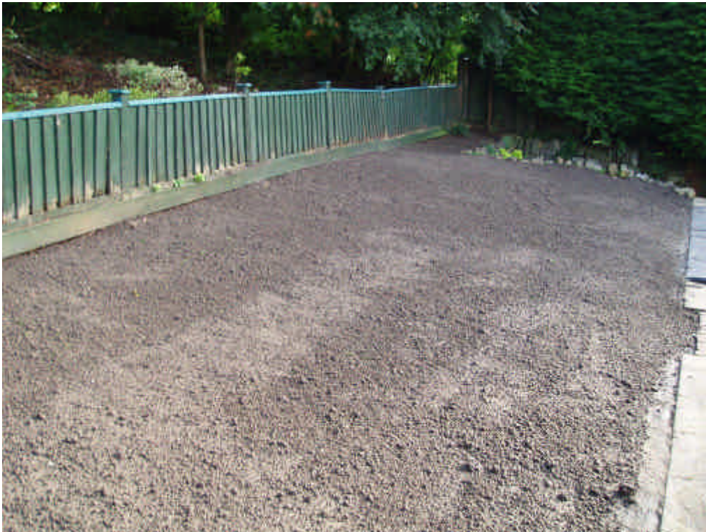
Photograph 7: Beech Cottage raised garden area after backfill (August 2008)
