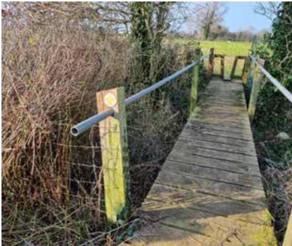
Recently cleared footpath bridge over ditch
