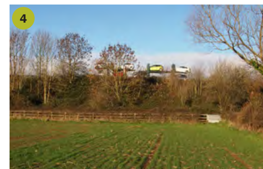
View of M5 and embankment on the north-east boundary
