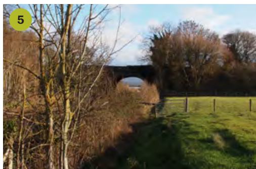
Great Western rail line and A4135 road bridge
