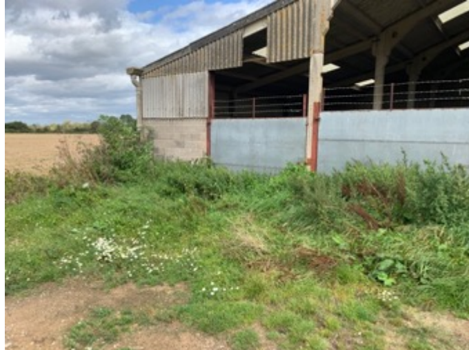
Photograph 50: Tall ruderal surrounding farm building.
