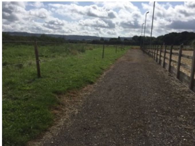
Photograph 47: Fencing surrounding the arena and paddocks.
