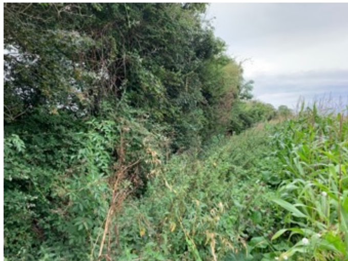
Photograph 67: Dry ditch along south hedgerow.
