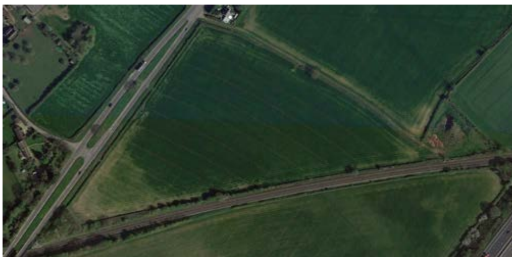
Figure 3: Field A aerial view.
