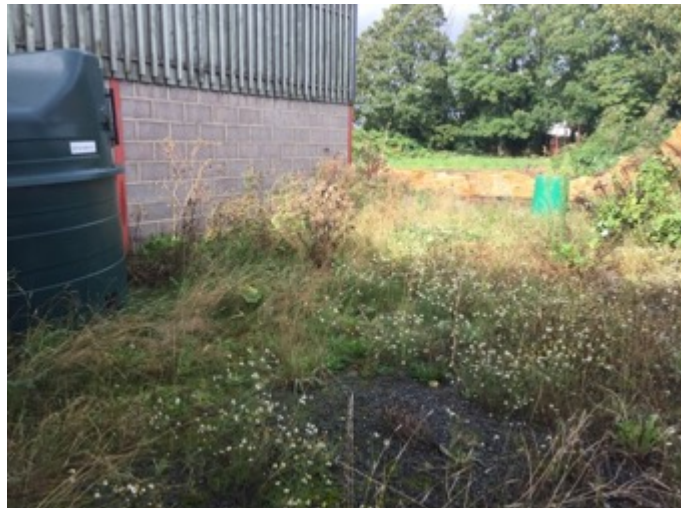
Photograph 43: Ephemeral/short perennial vegetation colonising around the buildings.
