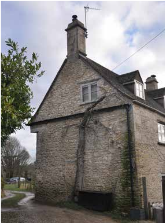
Old farm cottage with chamfered corner to give loaded hay carts access in Tickmorend
