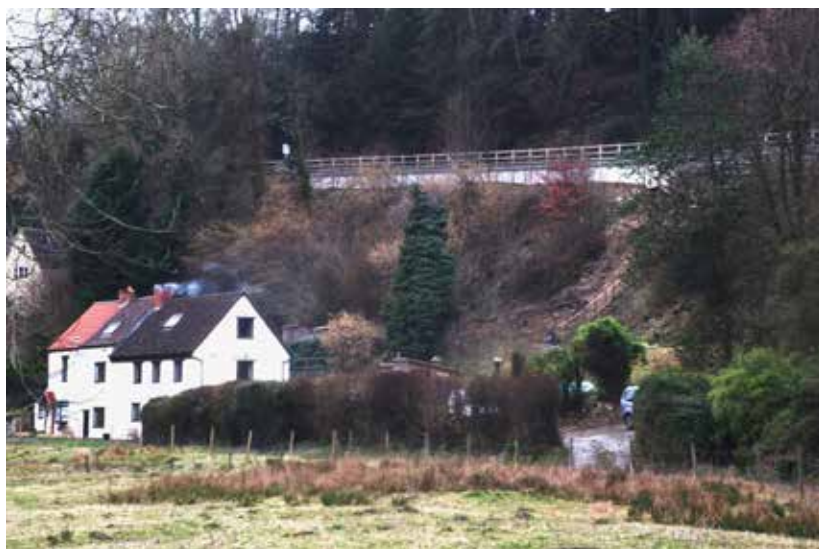
Part of the reconstructed B4058 roadway following collapse of the bank through subsidence
