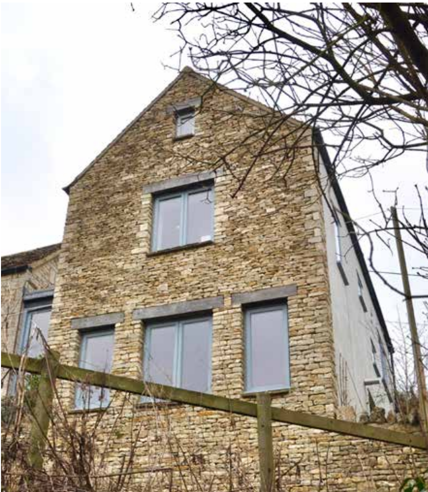
Contemporary extension to an old cottage with a well chosen natural stone finish that varies in tone and hue, and features timber lintels and well proportioned windows, Rockness
