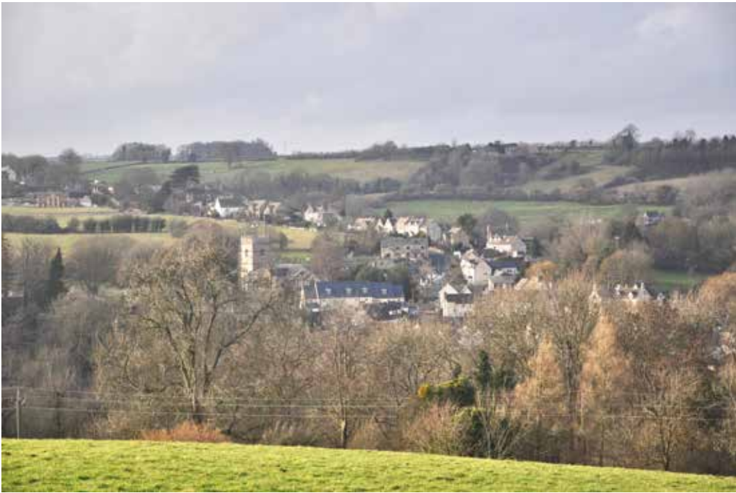
Horsley Village from footpath No. 46, showing the Parish Church and linear development along The Street. Incremental development since the 1930s, including a mid 20th Century council estate at Priory Fields and a recent, striking terrace by the Hog Inn, has been successfully absorbed into the landscape, hugging the lower contours. Views to the open countryside have been maintained
