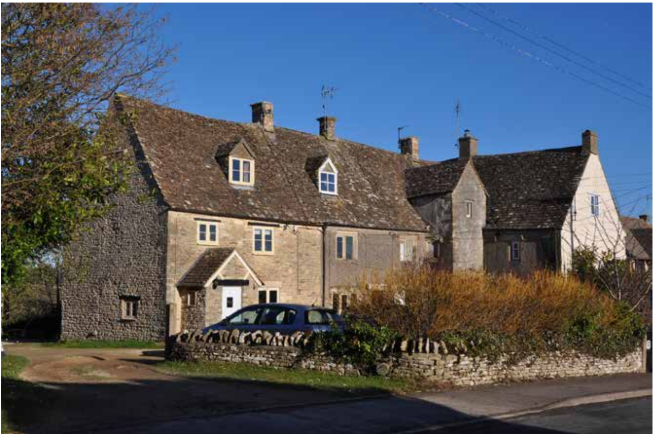
Park View Cottages. A listed early 17th Century farm building overlooking open countryside in Nupend, now divided into four dwellings. Features include a stair tower and a number of stone mullioned windows
