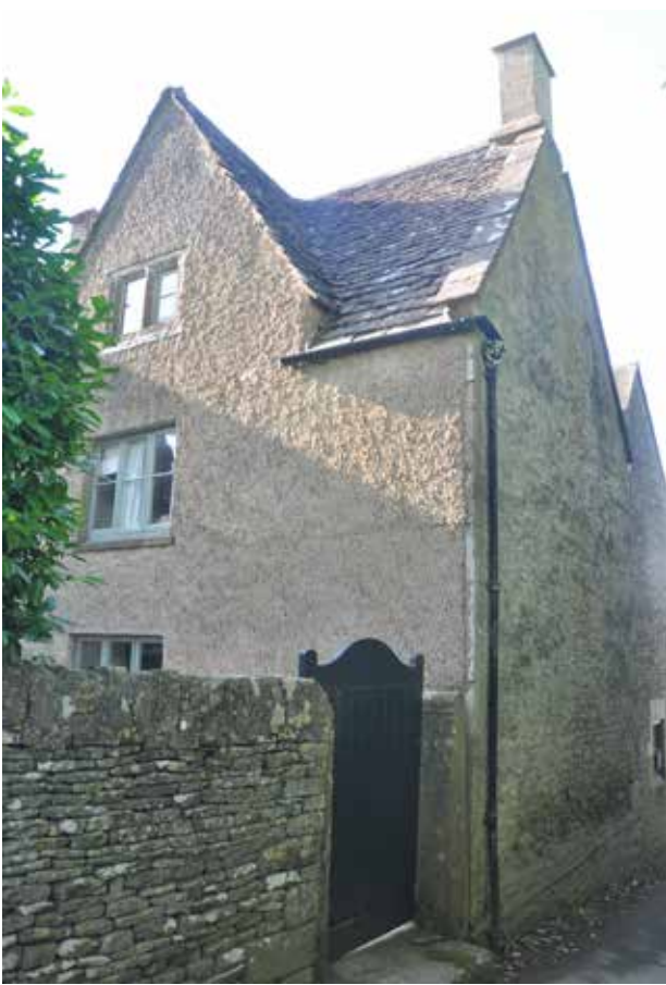
A listed mid 17th Century farmhouse at Upper Barton End with mullioned casement windows in stone and wood, rough cast render over rubble limestone, and Ashlar stone detail
