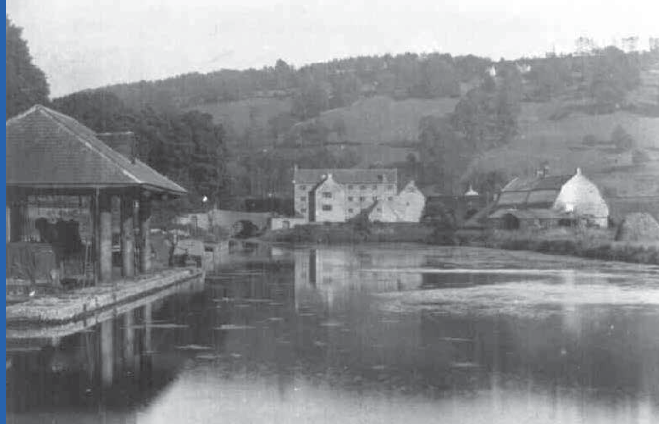
Brimscombe Basin from the North-west, early 1900's
