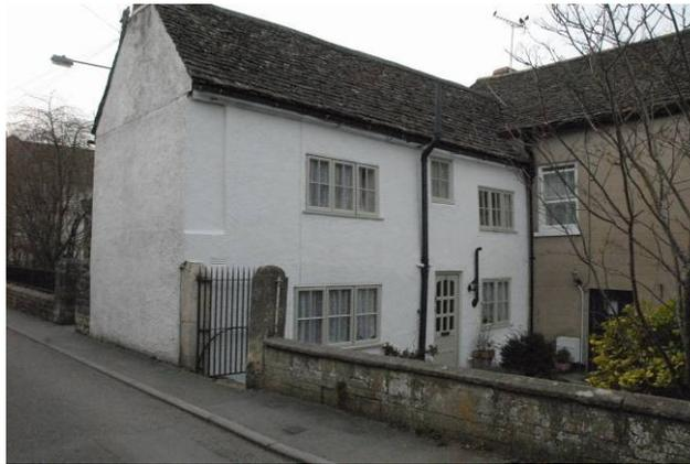
Two cottages in L-shape attached to Nos. 5 and 7 but not forming part of original Abbey Gate-house fabric. Probably C18. No. 9 is incised render, No. 11 in roughcast, both with Cotswold stone slate roof and brick stacks. L-shape, 2 storeys. No. 9 has 2 windows, plate glass sashes, one similar on ground floor and C20 door to left. No. 11 has 3 windows, 2 and 3-light wood casements, 2 to ground floor with central C20 half-glazed door.
