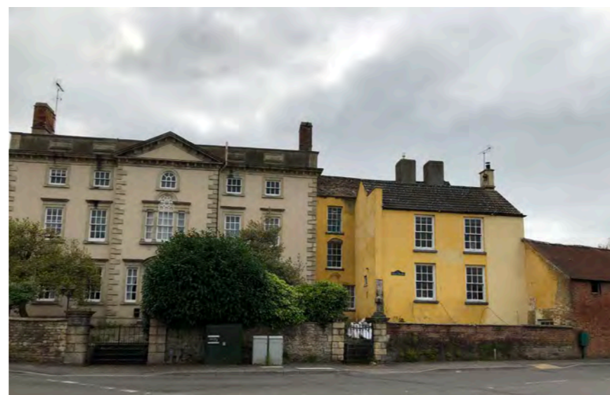
FIG. 11 GRADE II LISTED CHESTNUT PARK HOUSE, KINGSWOOD
